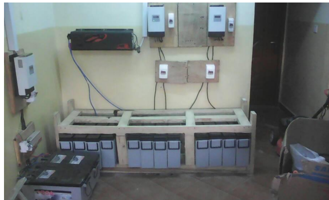
Figure 9. Arrangement of inverter, Charge Controller and Batteries
